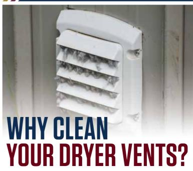
Many homes have flexible plastic or vinyl dryer vents that can cause a buildup of lint in the vent's ridges. Regular cleaning of your dryer vent can eliminate the risk of fire.
